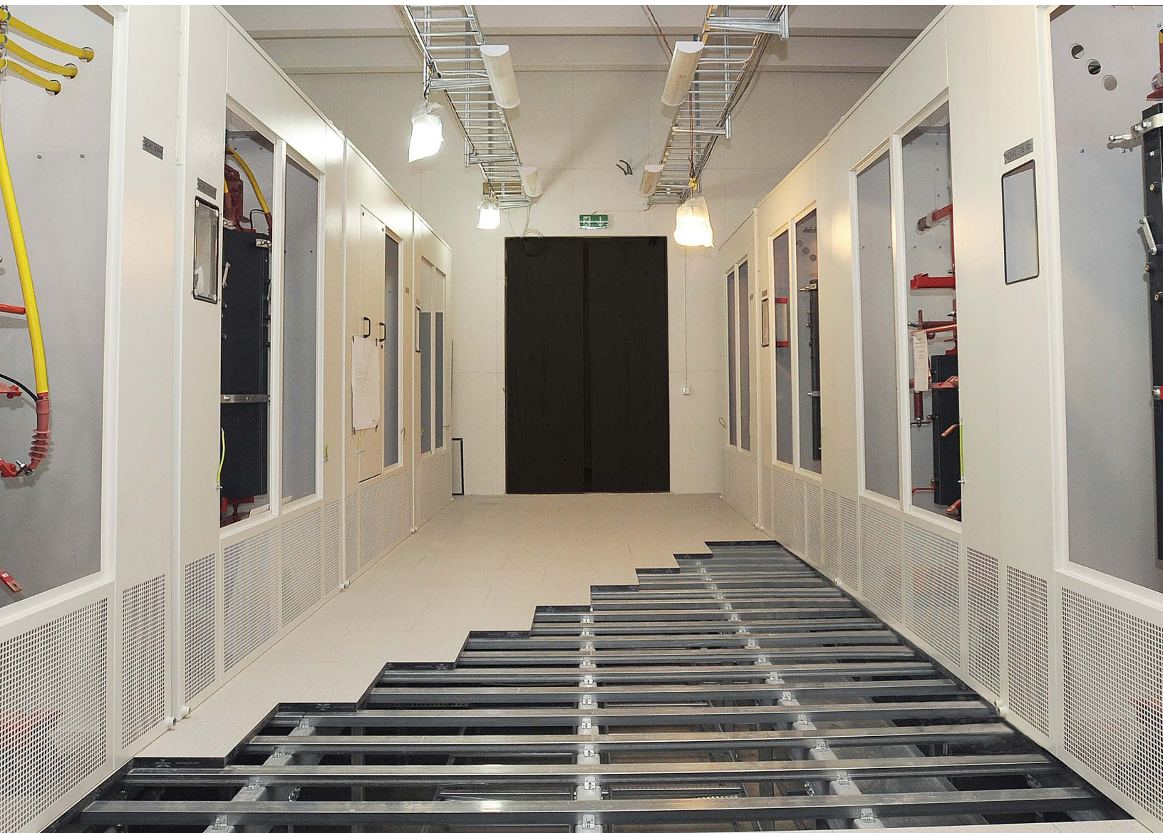
Transformer Room at Karolinska Hospital with reinforced Iso Floor Substructure supporting 16 Transformers with a total weight of 265,000 Lbs (120 ton).
