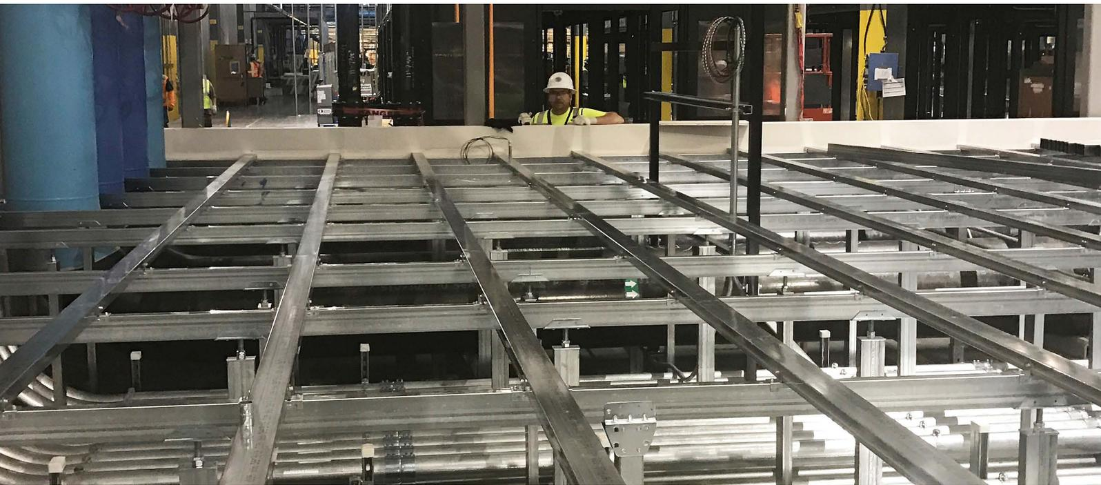
Iso Floor supporting 36.5 kN/m<sup>2</sup> of electrical equipment for a major technology company in Arizona.
