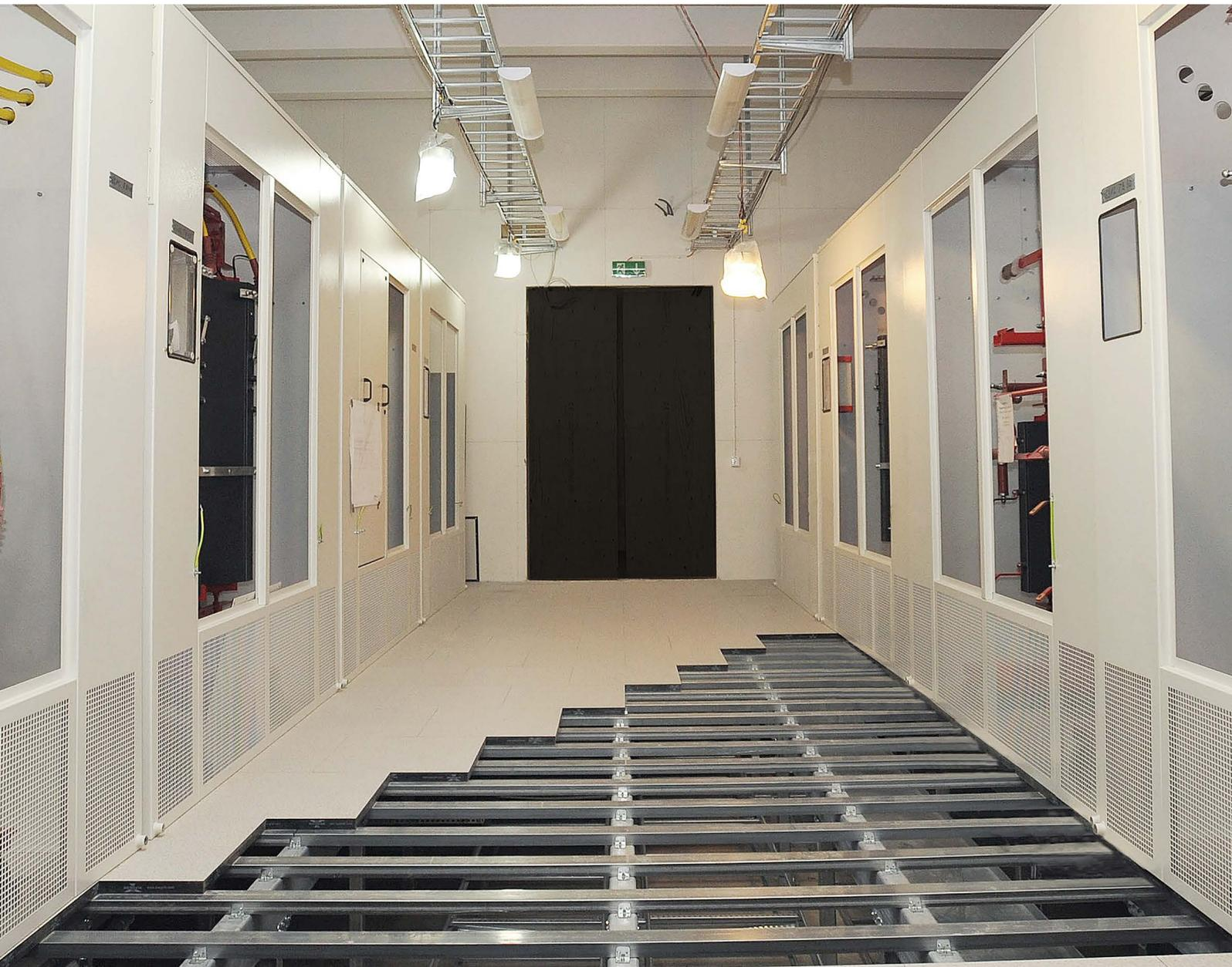
Transformer Room at Karolinska Hospital with reinforced Iso Floor Substructure supporting 16 Transformers with a total weight of 120 ton.
