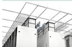
A load-bearing ceiling system that is both a dropped ceiling and a support grid in one cost effective solution.
