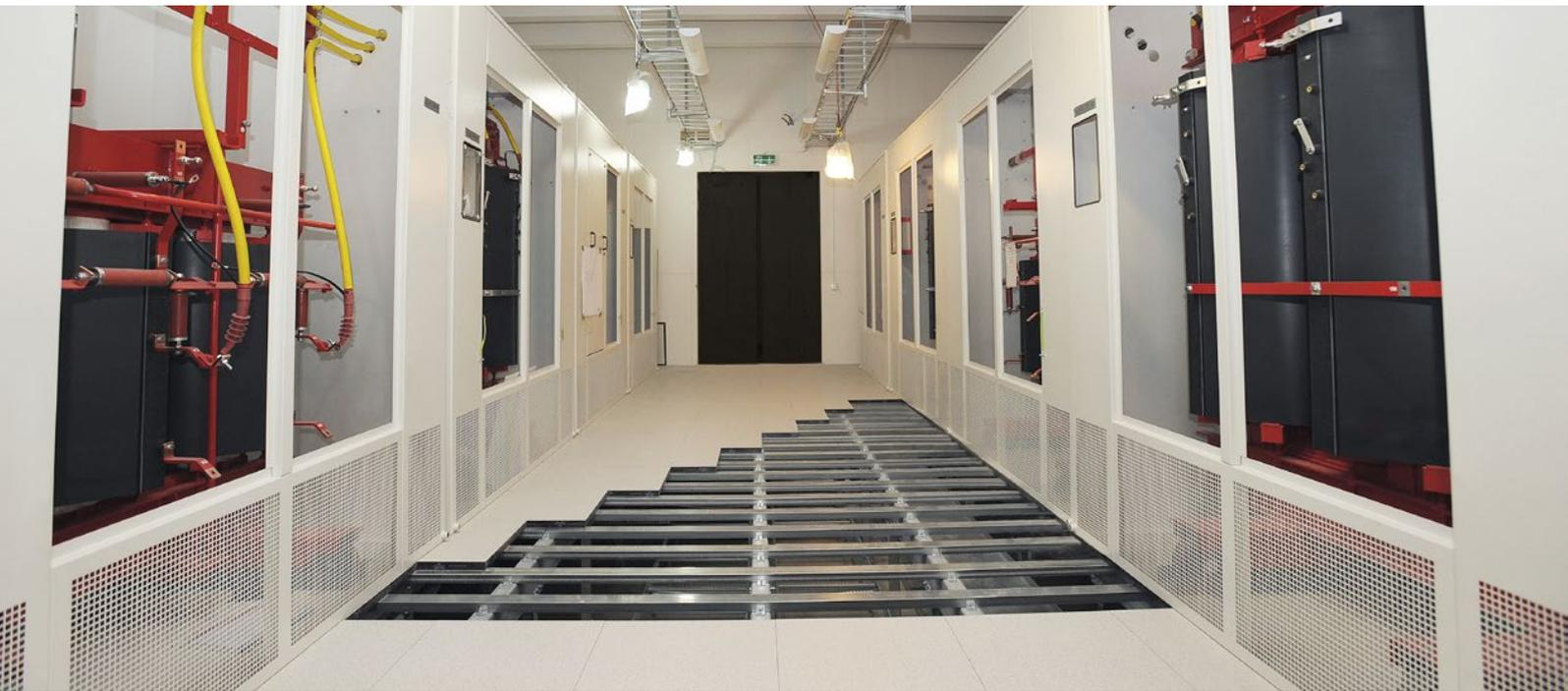
Transformer Room at Karolinska Hospital with reinforced Iso Floor Substructure supporting 16 Transformers with a total weight of 120 ton.
