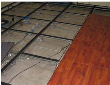
Existing floor structure is kept intact.
