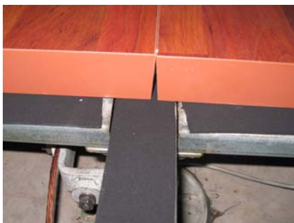
New rubber lining is glued to the structure.
