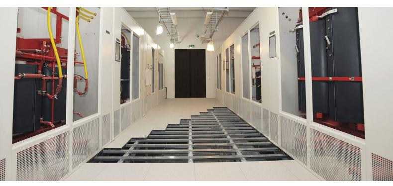
Transformer Room at Karolinska Hospital with reinforced Iso Floor Substructure supporting 16 Transformers with a total weight of 120 ton.
