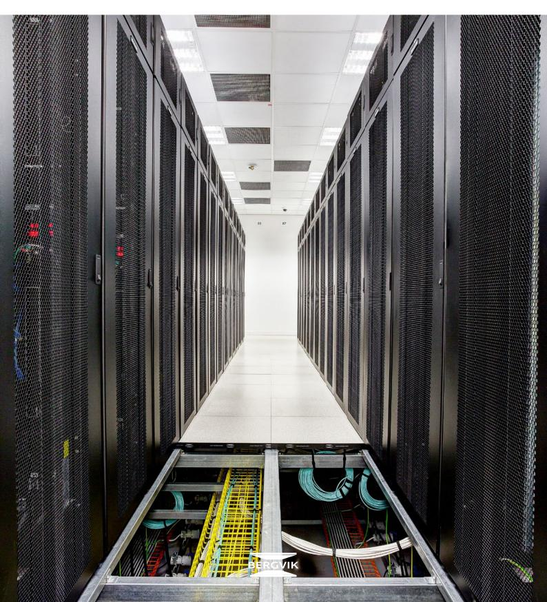
The Iso Floor system provides many added values for us, including maximum flexibility, stability and strength. By using the Bergvik floor we don't need separate equipment stands for heavy CRAC's, UPS's etc.
