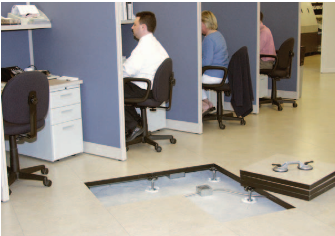
Tech Floor with linoleum panel finish at Taylor Bank, Berlin MD
